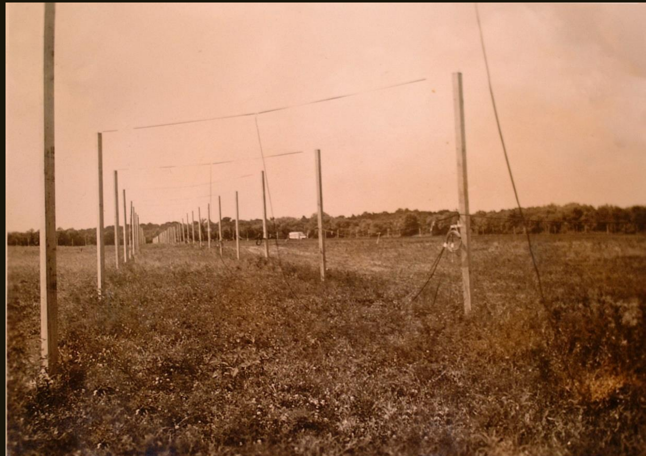
The 'Mills Cross Array' used by Burke and Franklin to detect radio emissions from Jupiter [1].
