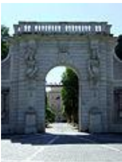
The entrance from outside the Villa
