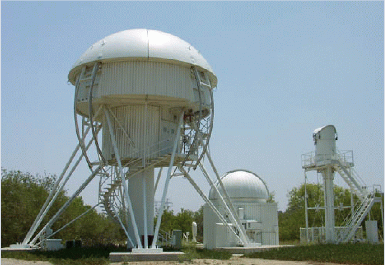
SFO after repairs following the Northridge Earthquake
